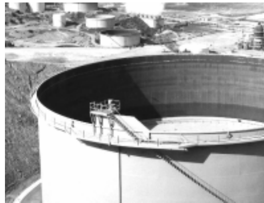
Figure E-6a—Open Top (External) Floating Roof Tank
