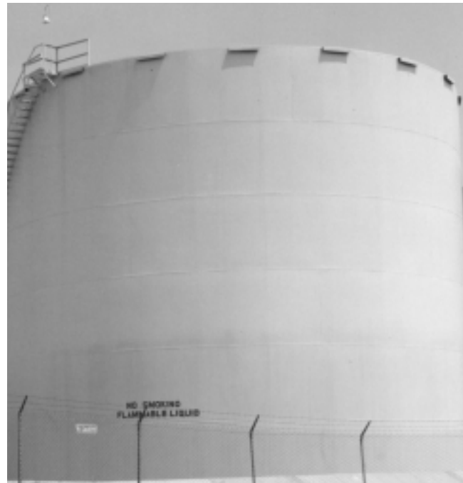
Figure E-5a—Internal (Covered) Floating Roof Tank
