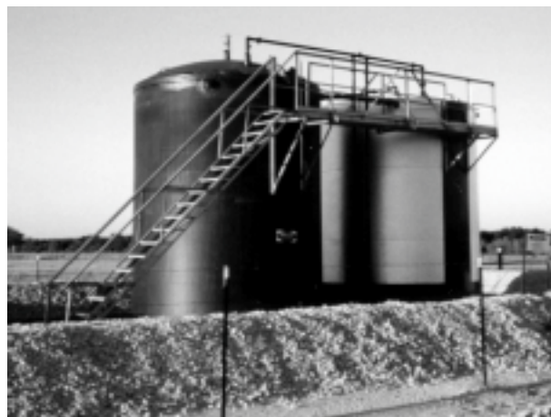
Figure E-2—Low-Pressure Tanks without Weak Seam
