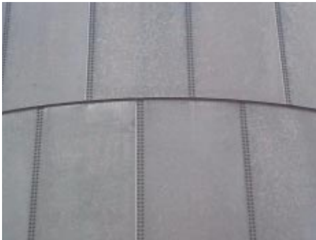
Figure E-4—Close-up View of Bolted Tank Seams
