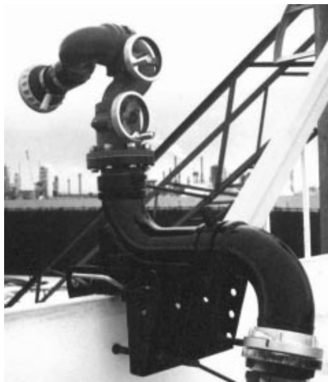
Figure 14—Special Portable Monitor Attached to Edge of Floating Tank Roof to Fight Rim Seal Fires
